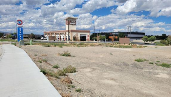
Car Wash Looking northwest from Patterson Rd
