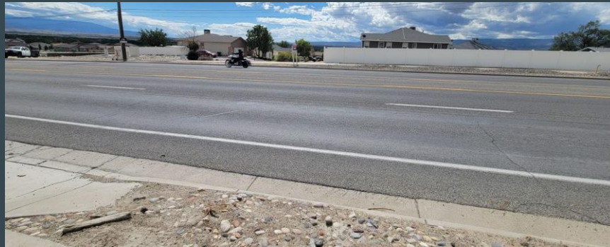
Patterson Rd Looking south from the site
