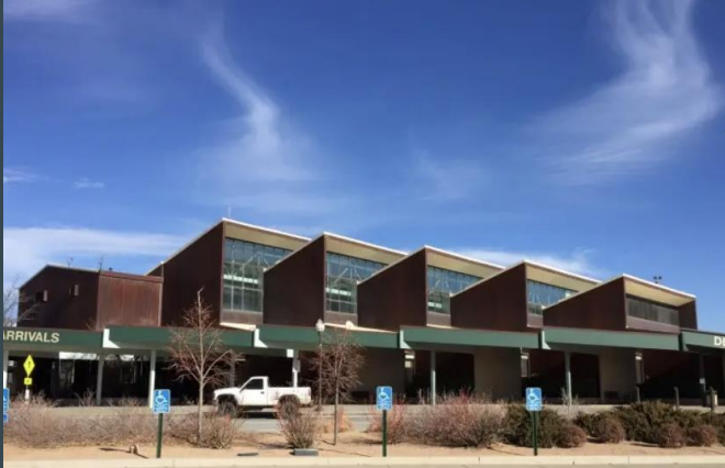
Grand Junction Airport
